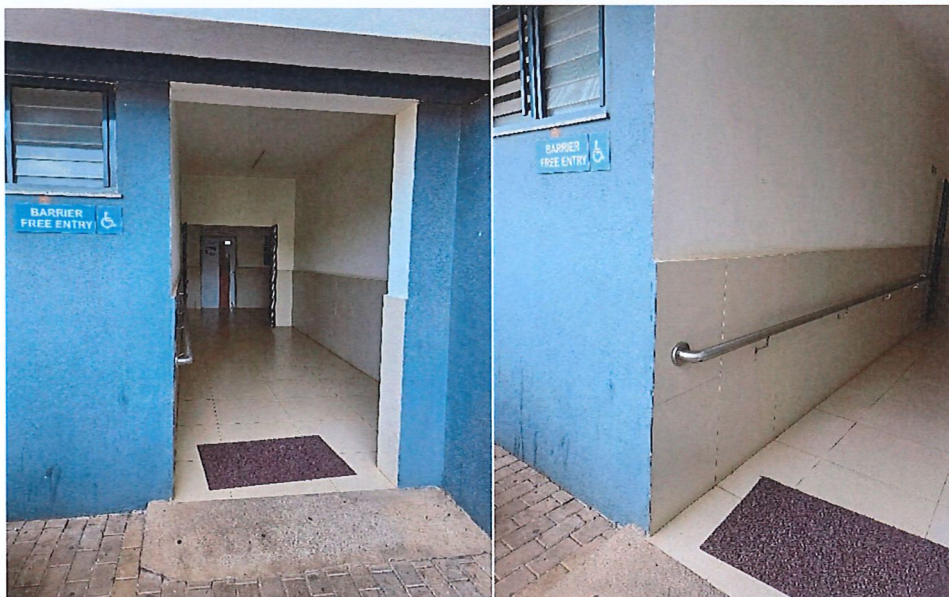
Barrier free entry with railings attached
