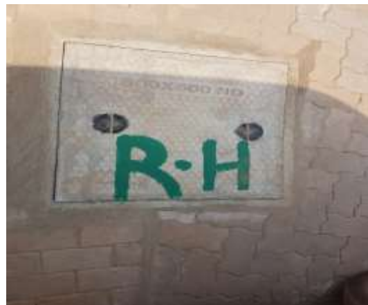
Figure 2 Rain Water Manhole Covering of the Tank
