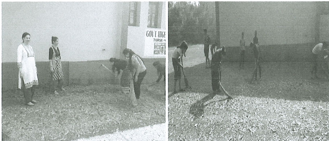
Cleaning of Government High School, Torxem School Premises
